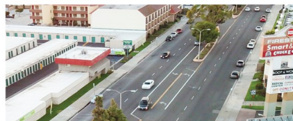
Firestone Boulevard Widening, Norwalk
